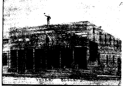
Construction of Yoder Garage
