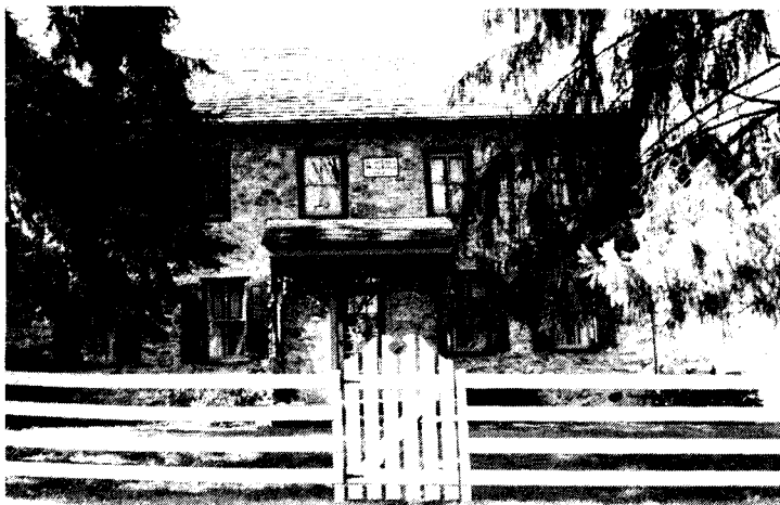
This is a front view of the newest of the three buildings shown in the previous photograph. The property is on the road from Lobachsville to New Jerusalem, PA. The stone over the doorway says "Jacob Yoder, Mary Yoder, 1829" (which apparently is the date it was constructed). This building, now the main residence, has a wood shingle roof (unlike the other buildings which all have "Oley tile" roofs).
