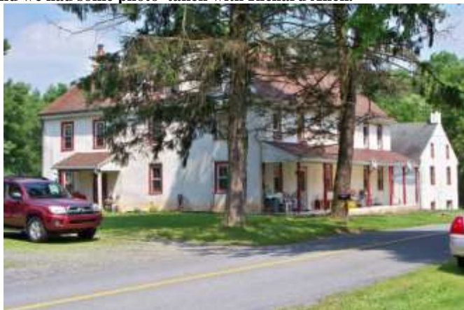
MAIN HOUSE WITH ITINERANT HOUSE BEHIND
