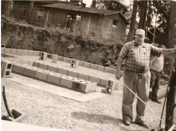
Building Supervisor Kenneth L. Yoder Measures the Footer
